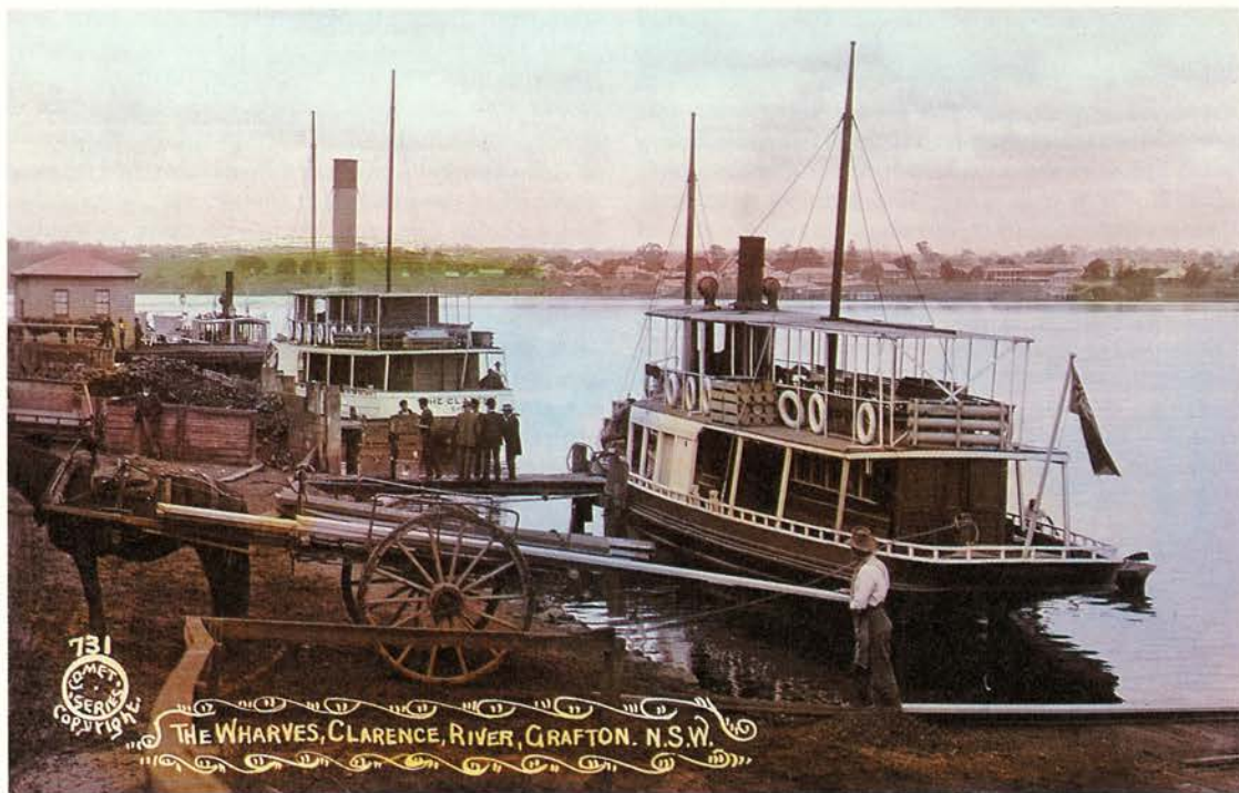
Small river steamers on the Clarence River, Grafton, New South Wales. Such vessels provided vital links until largely replaced by road and railway bridges. Postcard, c1900.
